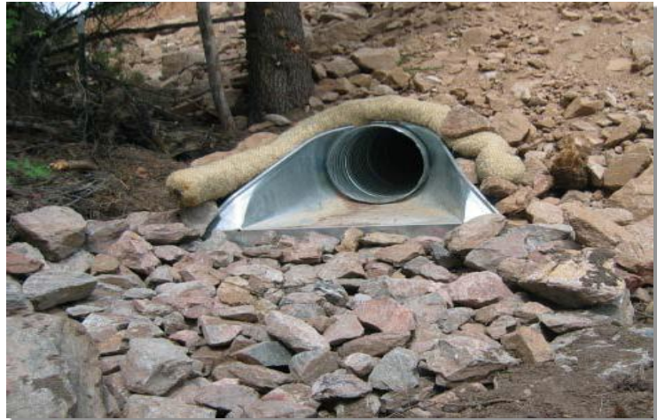
Photograph TOP-1. Riprap outlet protection.
