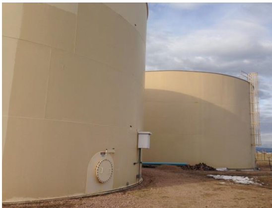
Figure 6: PBHMD 1 MG Water Storage Tank (left) and 0.5 MG Water Storage Tank (Right)
