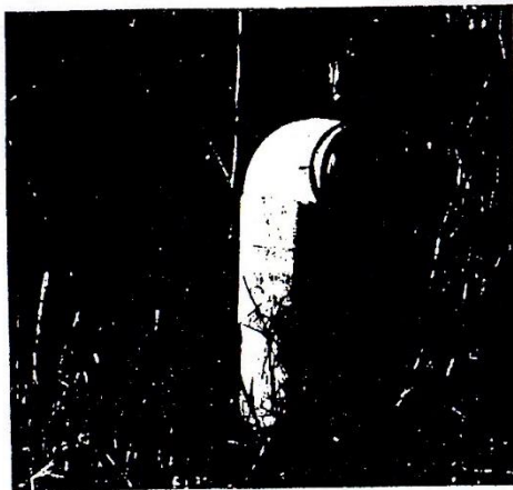
Figure B-5-1(a) Dry hydrant.
