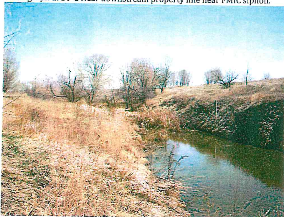
Photograph 2: DP2 Near old ranch road crossings.
