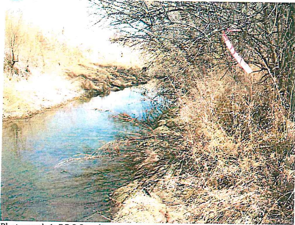
Photograph 1: DP 3 Standing water in channel bed.
