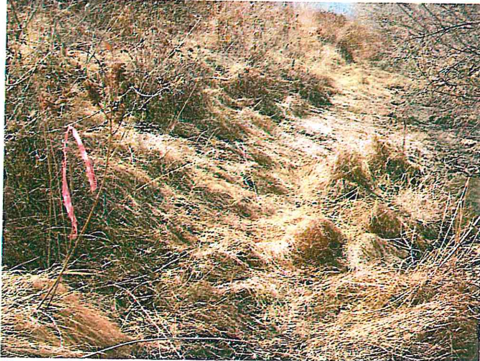
Photograph 2: DP4 Located downstream of existing trapezoidal channel.
