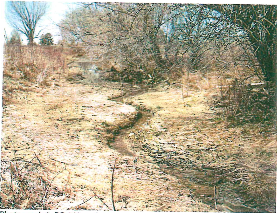
Photograph 1: DP 1 Near downstream property line near FMIC siphon.
