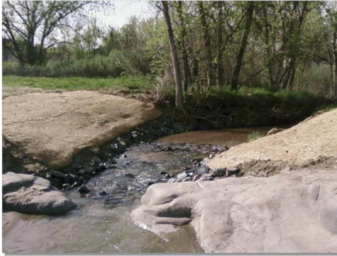
Photograph SS-1. Streambank stabilization using geotextiles following installation of a permanent in-stream grade control structure.
