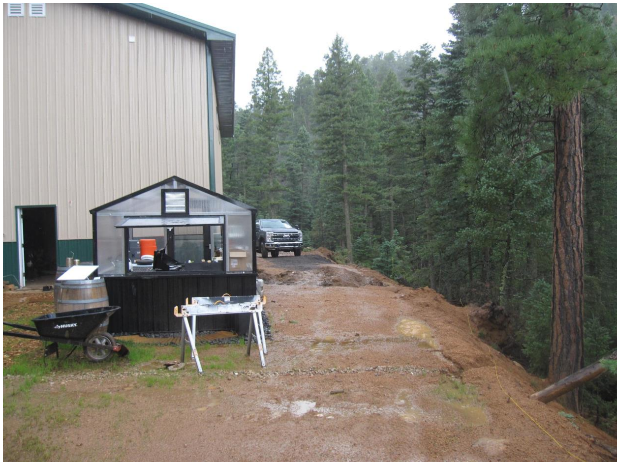
Photo 6. View along the south side of the garage structure. The distance to the tree line ranges from 15 – 16 feet.
