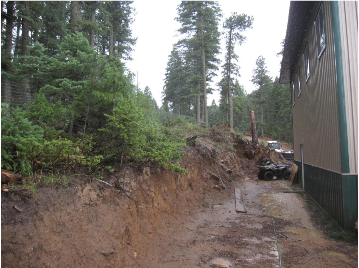
Photo 7. This represents the view from the northeast corner of the garage forward to the northwest corner. Additional trees uphill from the structure are being removed to prevent flames from touching the structure.
