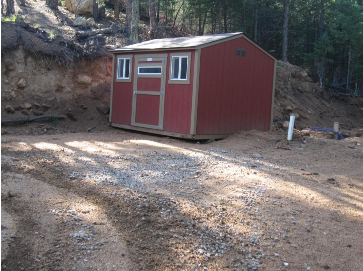
Photo 4. A view of the Tough Shed. Note the positioning on and around the non-flammable soil surface.
