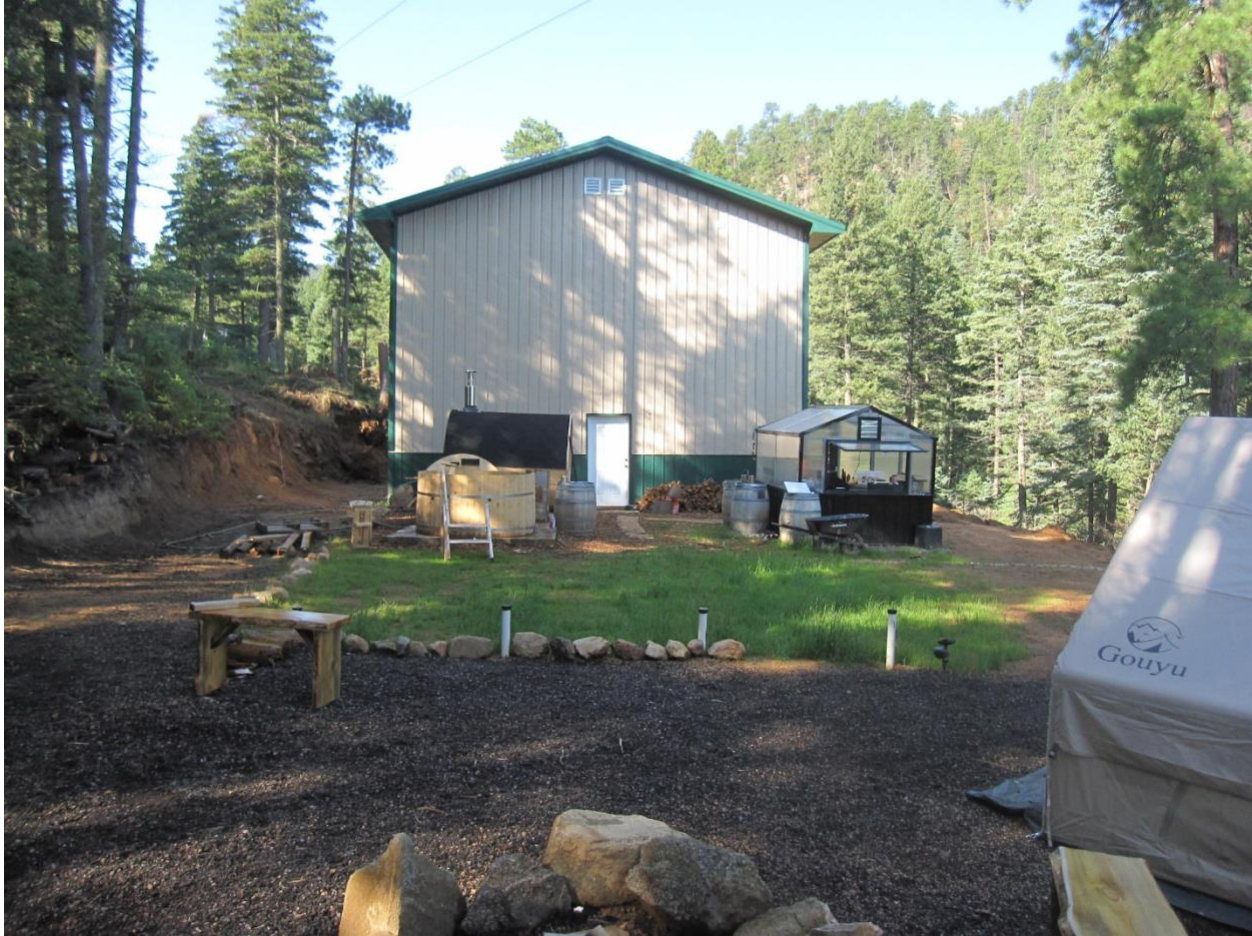
Photo 5. The view from the east edge of the living space back towards the garage. The distance is approximately 75 feet. This would represent Zone 1 (5-30 feet) & 2 (30-100 feet) as it relates to Defensible Space
