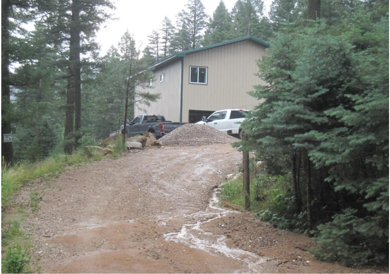
Photo 1. View of Garage structure from the lower end of the driveway. The west and south exterior walls can be reached well within the 150-foot requirement (6.3.4 B. General, 3 Access to Structures. ii.).
