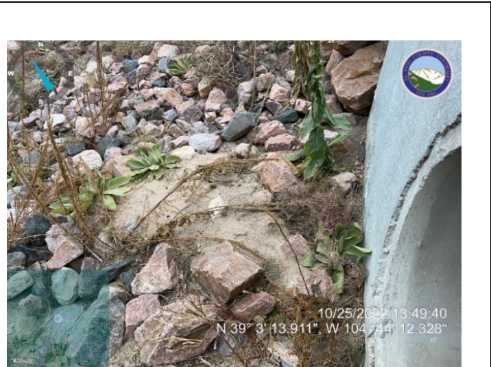
Photo 2: Remove sediment from riprap pad, southwest of culvert at STA. 46+70.97.
