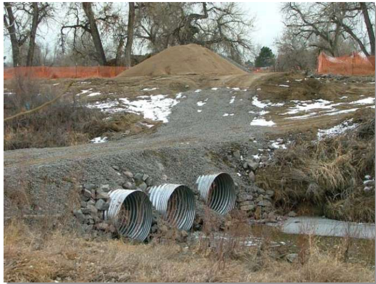
Photograph TSC-1. A temporary stream crossing using culverts. Photo courtesy of Tom Gore.
