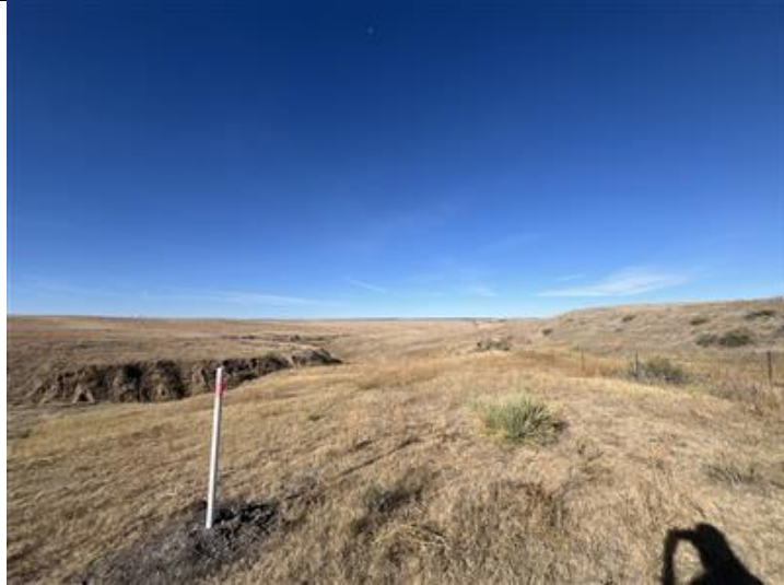
18. STR 428 – Facing W.
