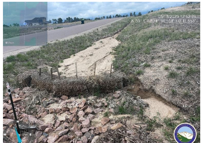
Photo 4: Regrade and stabilize ditches along Ward Lane. Remove sediment from riprap and implement as per approved plans.
