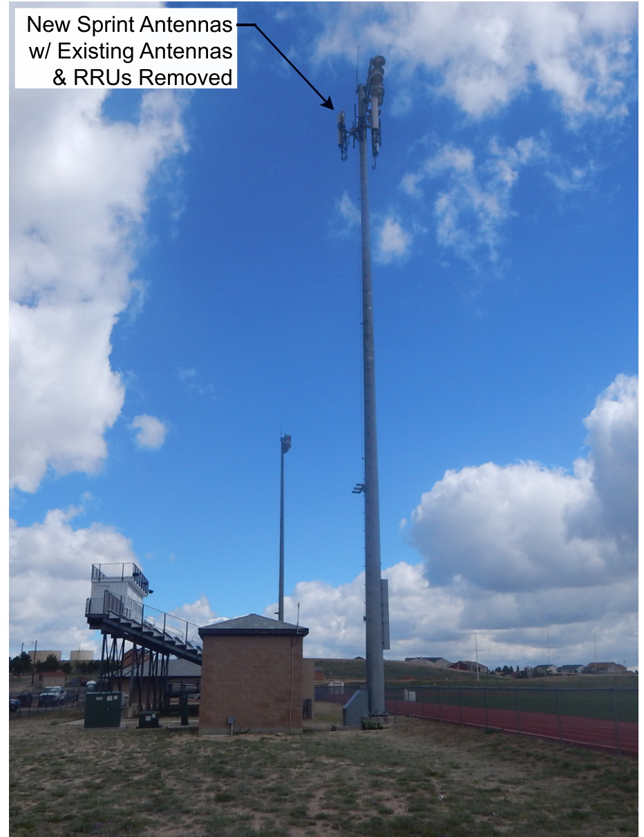
New View from the South
