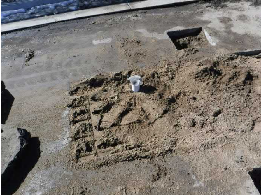
Percolation Test Location P-1
