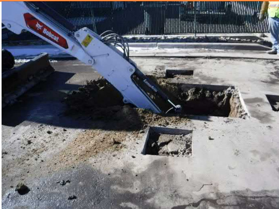
Test Pit During Excavation
