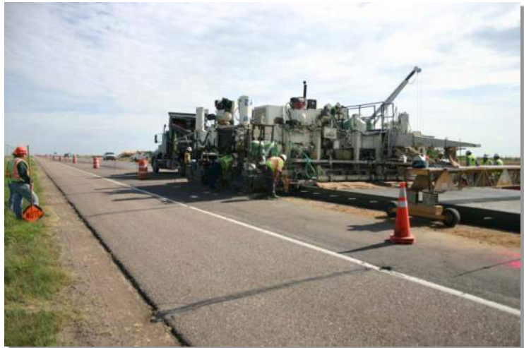
Photograph PGO-1. Paving operations on a Colorado highway. Photo courtesy of CDOT.
