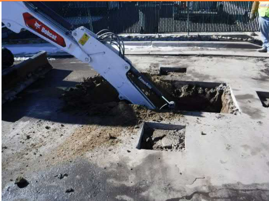
Test Pit During Excavation
