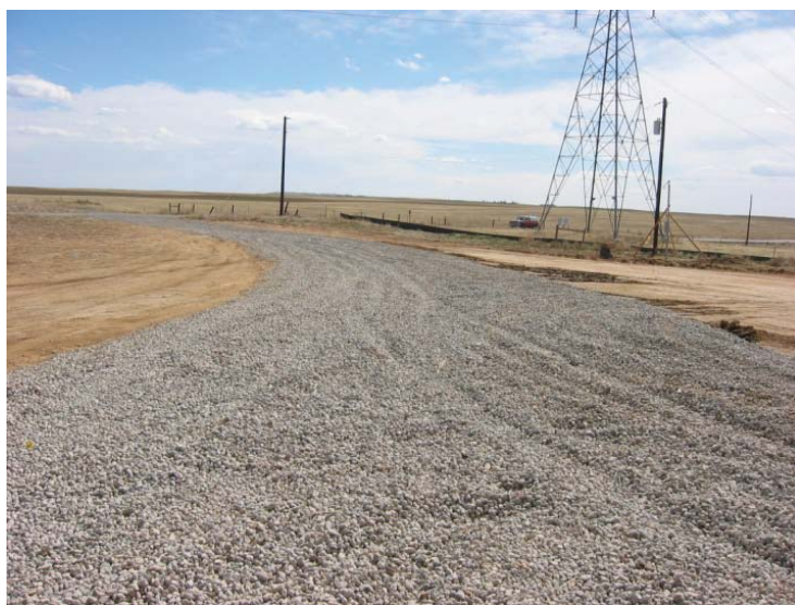
Photograph SCR-1. Stabilized construction roadway.
