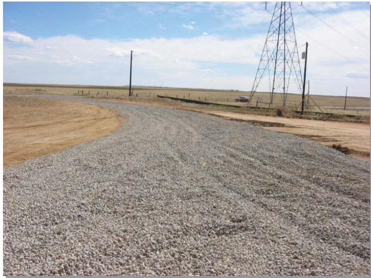
Photograph SCR-1. Stabilized construction roadway.
