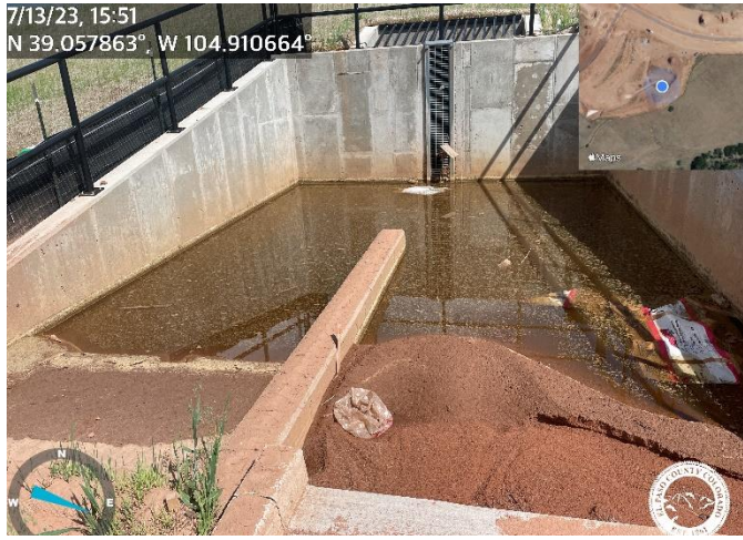
Photo 3: Remove sediment from outlet structure and remove debris from well screen.
