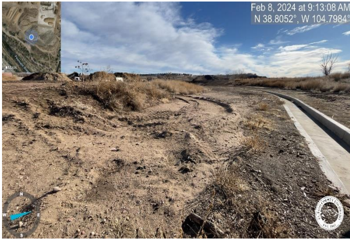
Photo 5: Fine grade pond bottom to match the approved grade.
