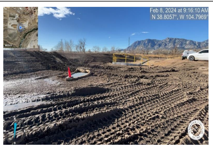
Photo 4: Flow currently bypasses inlet behind the east forebay. Regrade to promote flow into type D inlet.
