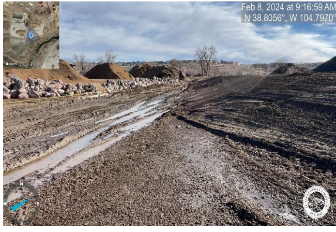
Photo 8: East of Pond: Fine grade drainage to pond to promote positive drainage (remove ruts).
