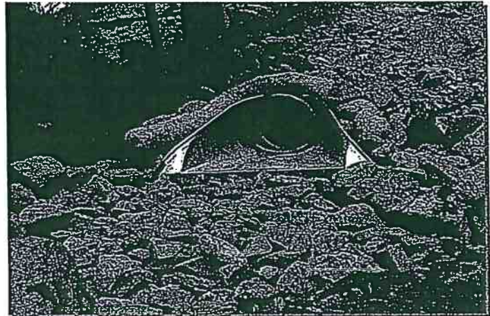
Photograph TOP-1. Riprap outlet protection.
