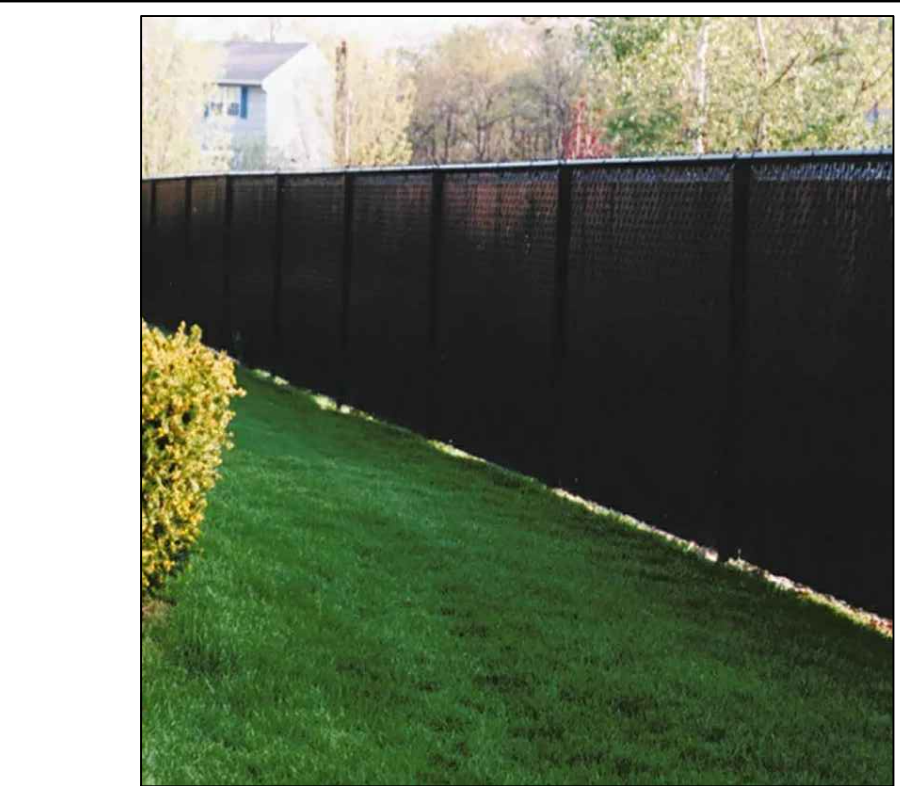
F CHAIN LINK FENCE WITH SLATS NOT TO SCALE
