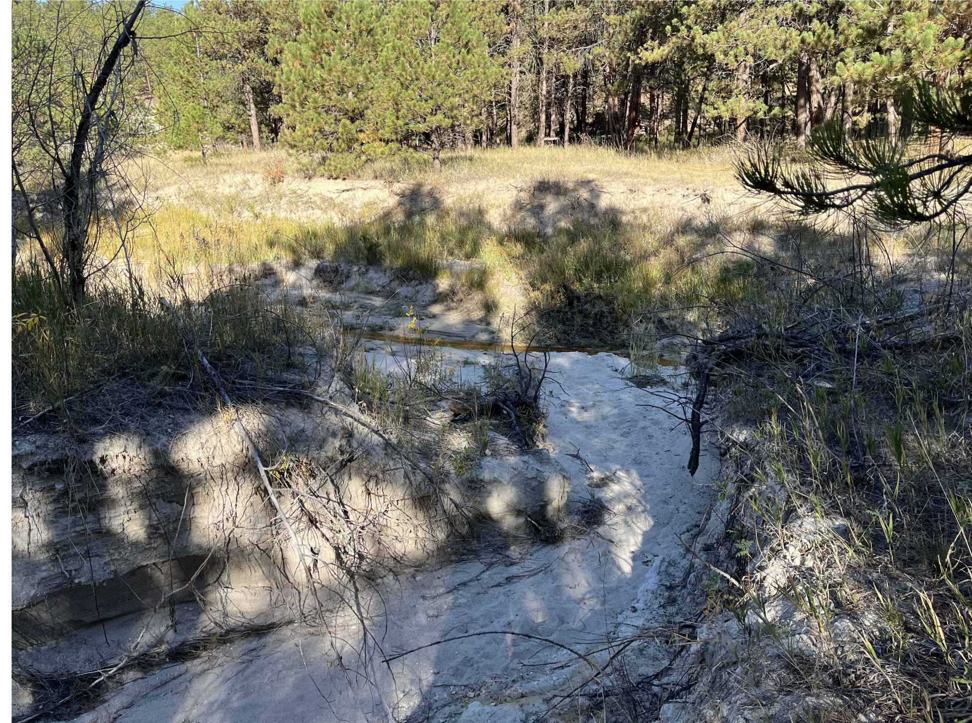
13. EXISTING DRAINAGE PATH 3 AT CONFLUENCE WITH KETTLE CREEK
