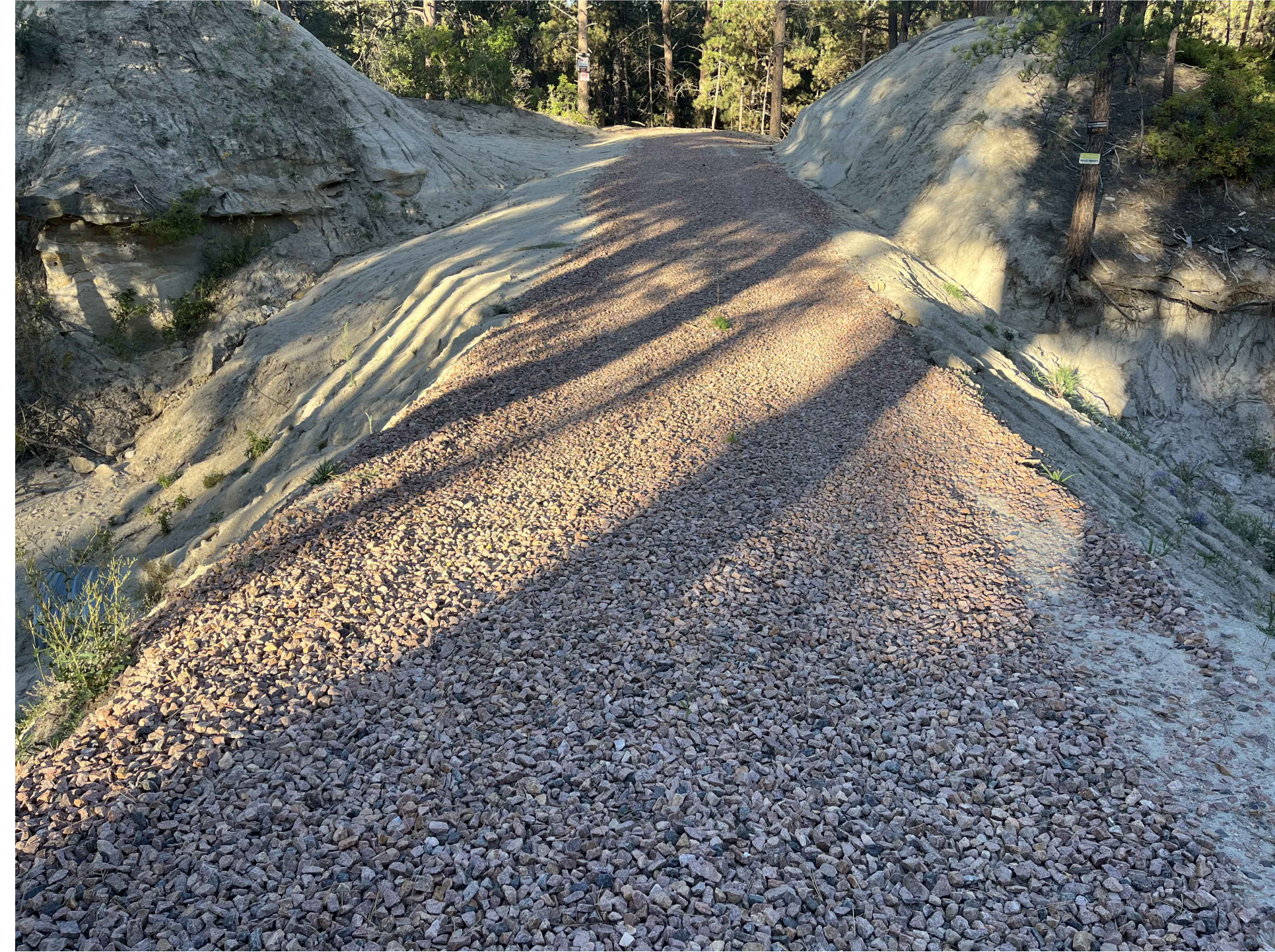
1. EXISTING 48' RCP CULVERT FROM ROAD
