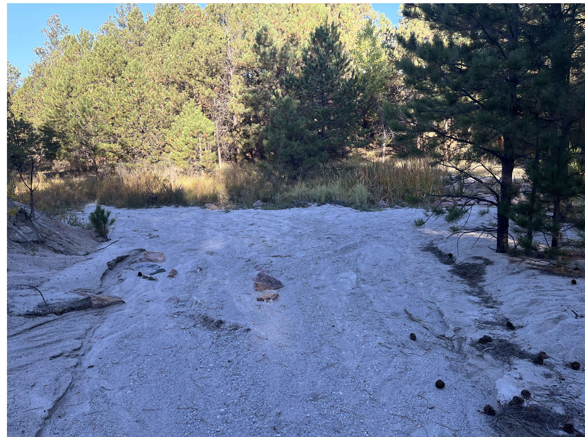
10. EXISTING DRAINAGE PATH 2 AT CONFLUENCE WITH KETTLE CREEK
