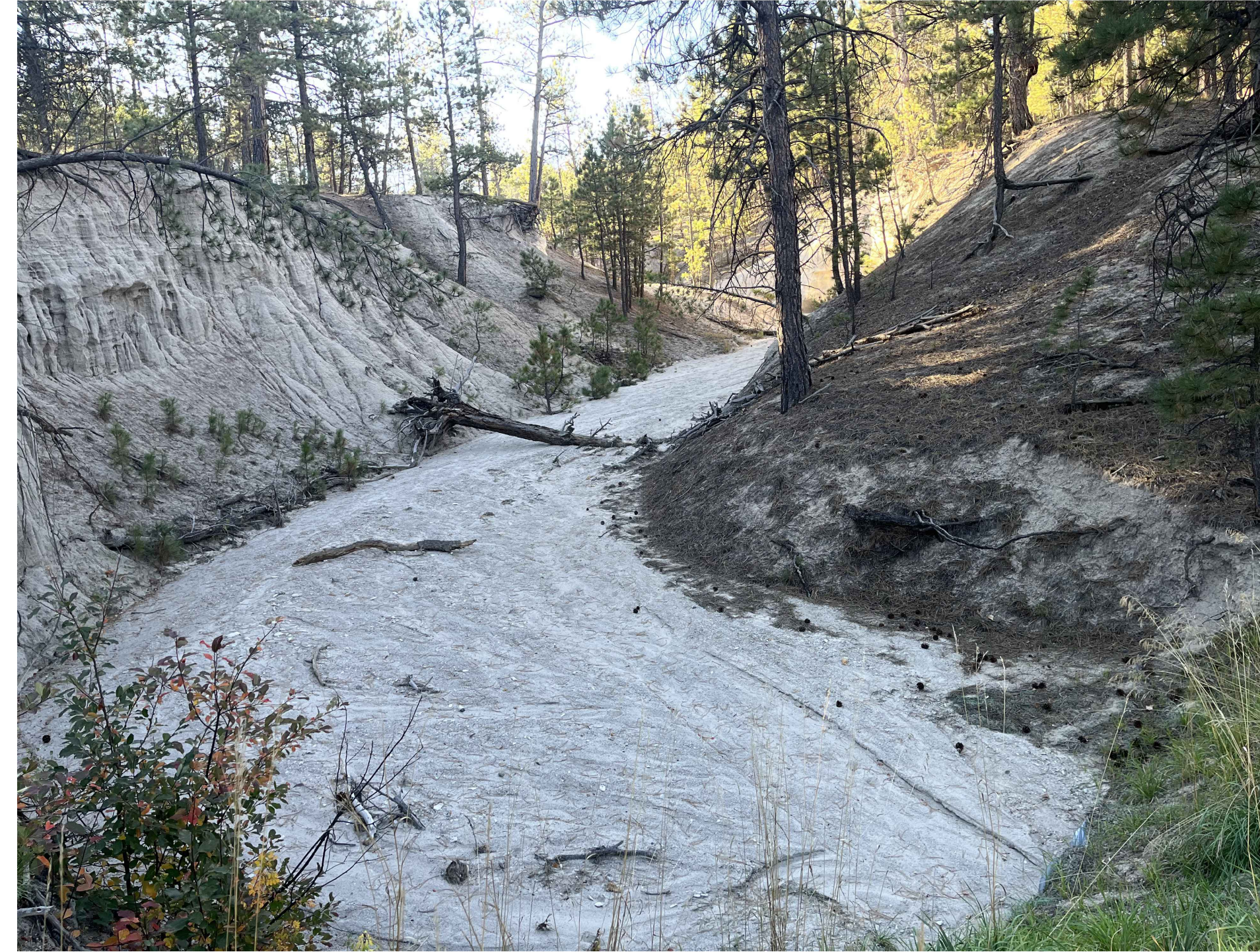
8. EXISTING TRIPLE 24' RCP CULVERT-UPSTREAM
