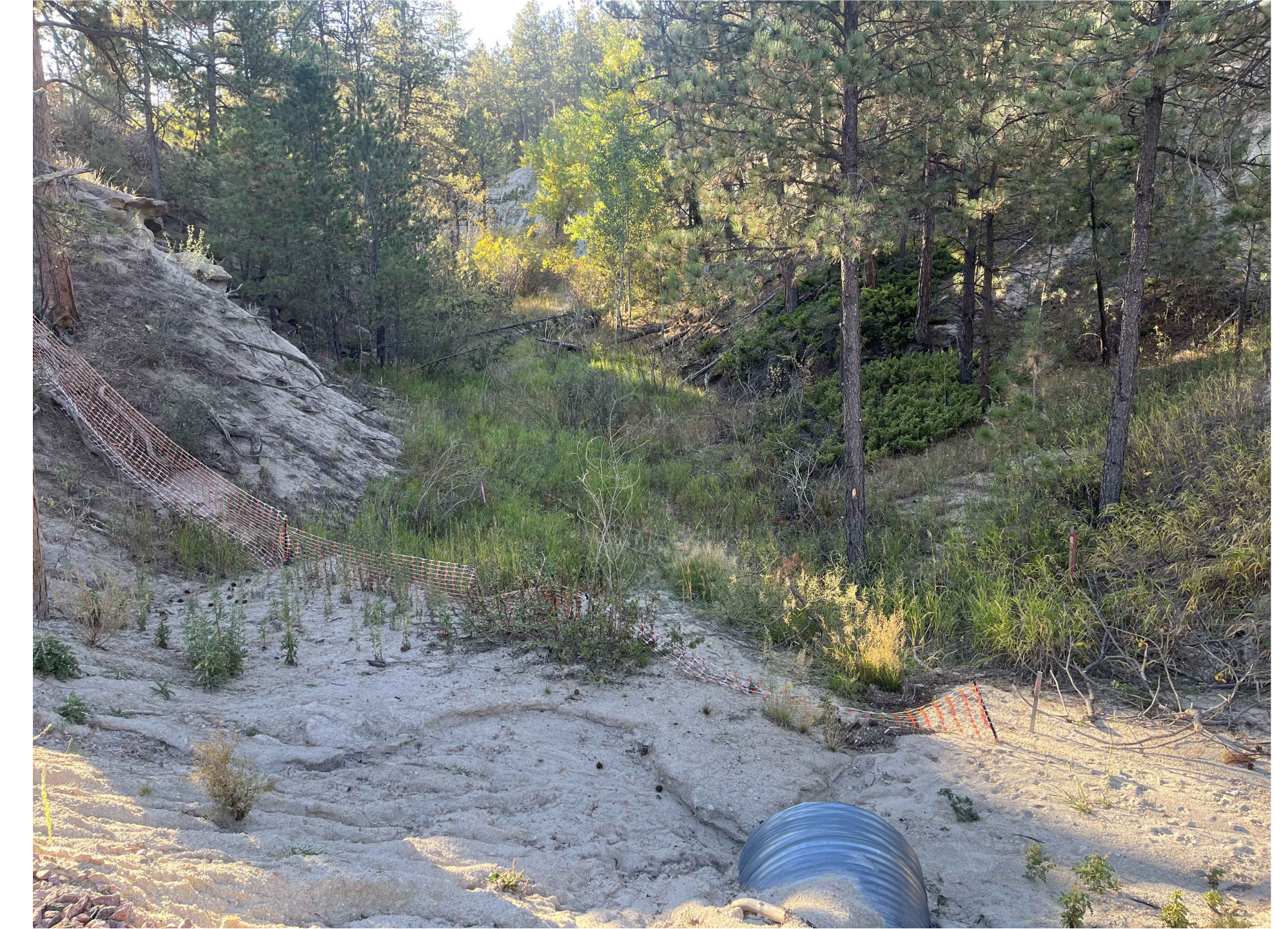
3. EXISTING 48' RCP CULVERT-UPSTREAM
