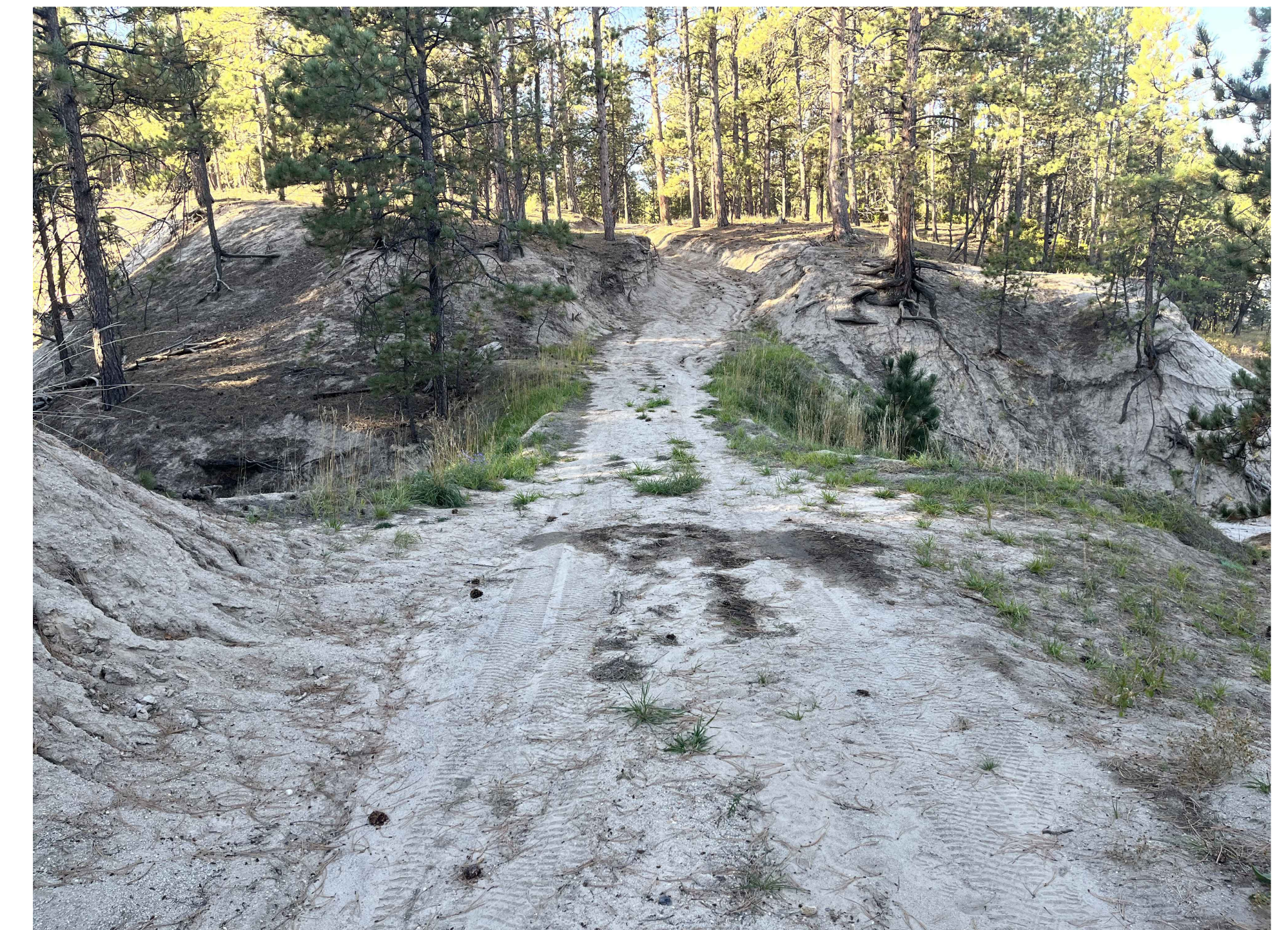
6. EXISTING TRIPLE 24' RCP CULVERT FROM ROAD
