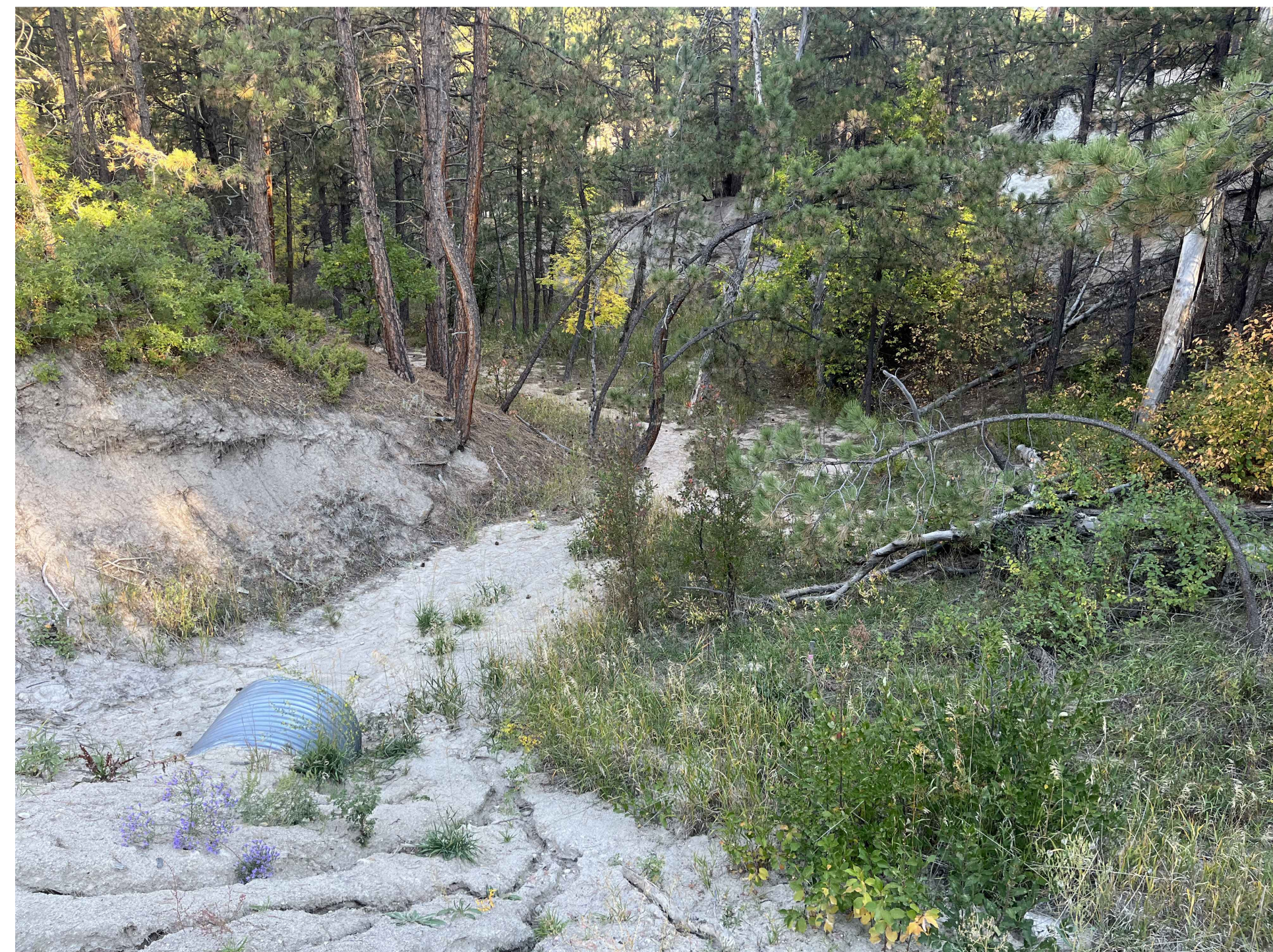
4. EXISTING 48' RCP CULVERT-DOWNSTREAM
