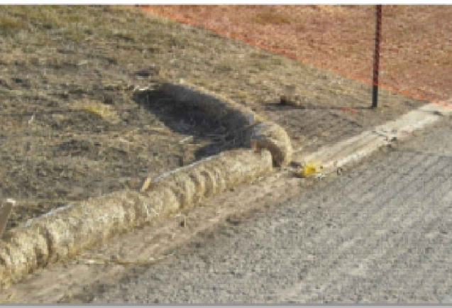
Photographs SCL-1 and SCL-2. Sediment control logs used as 1) a perimeter control around a soil stockpile, and, 2) as a "J-hook" perimeter control at the corner of a construction site.
