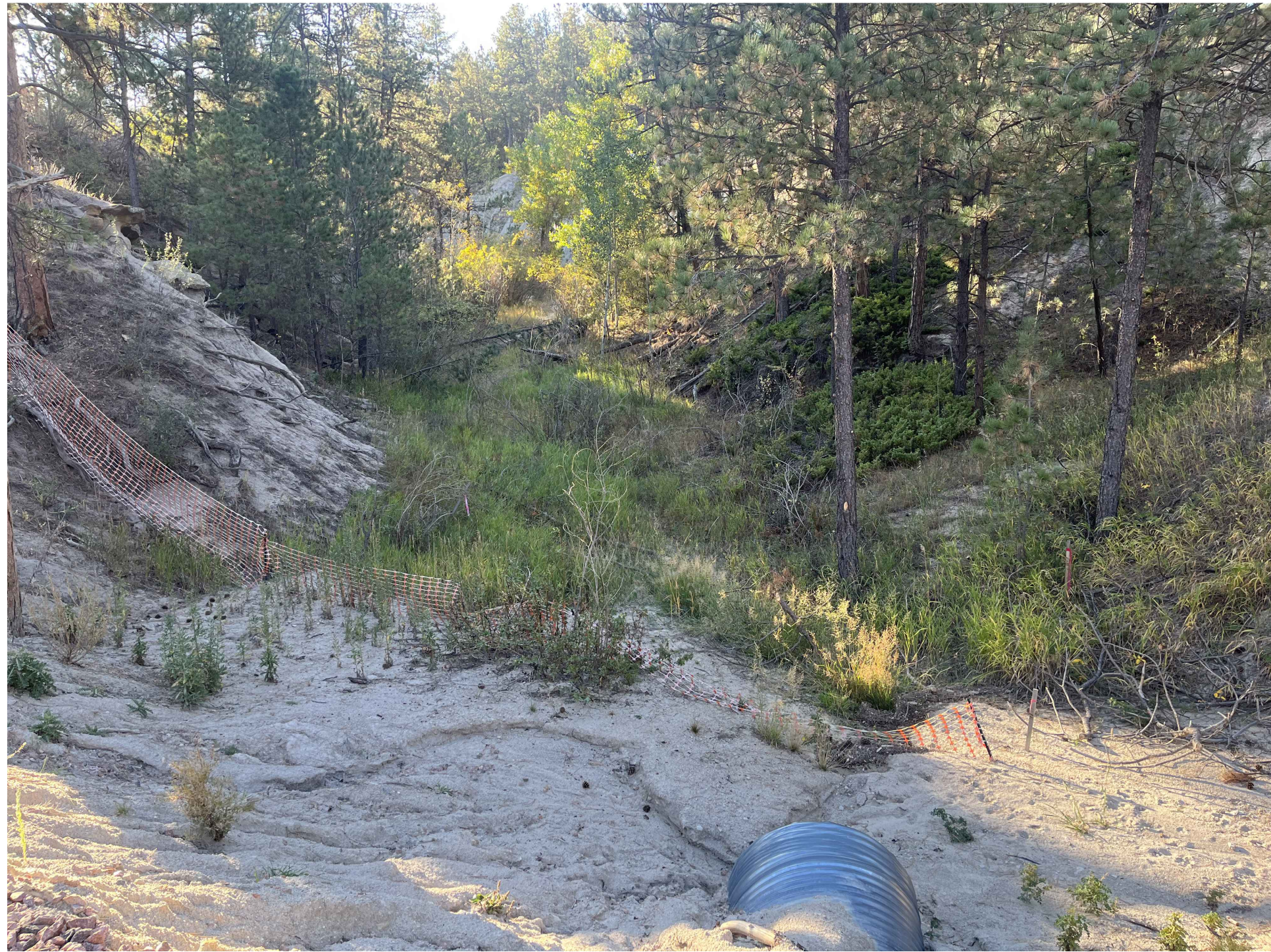
3. EXISTING 48" RCP CULVERT-UPSTREAM
