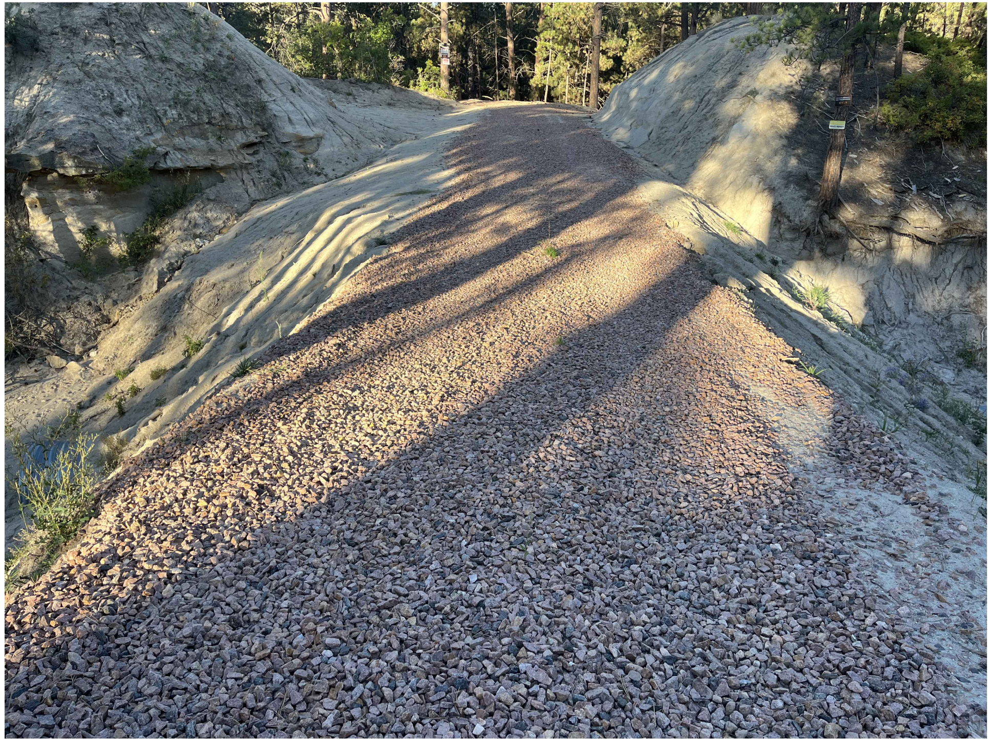
1. EXISTING 48" RCP CULVERT FROM ROAD
