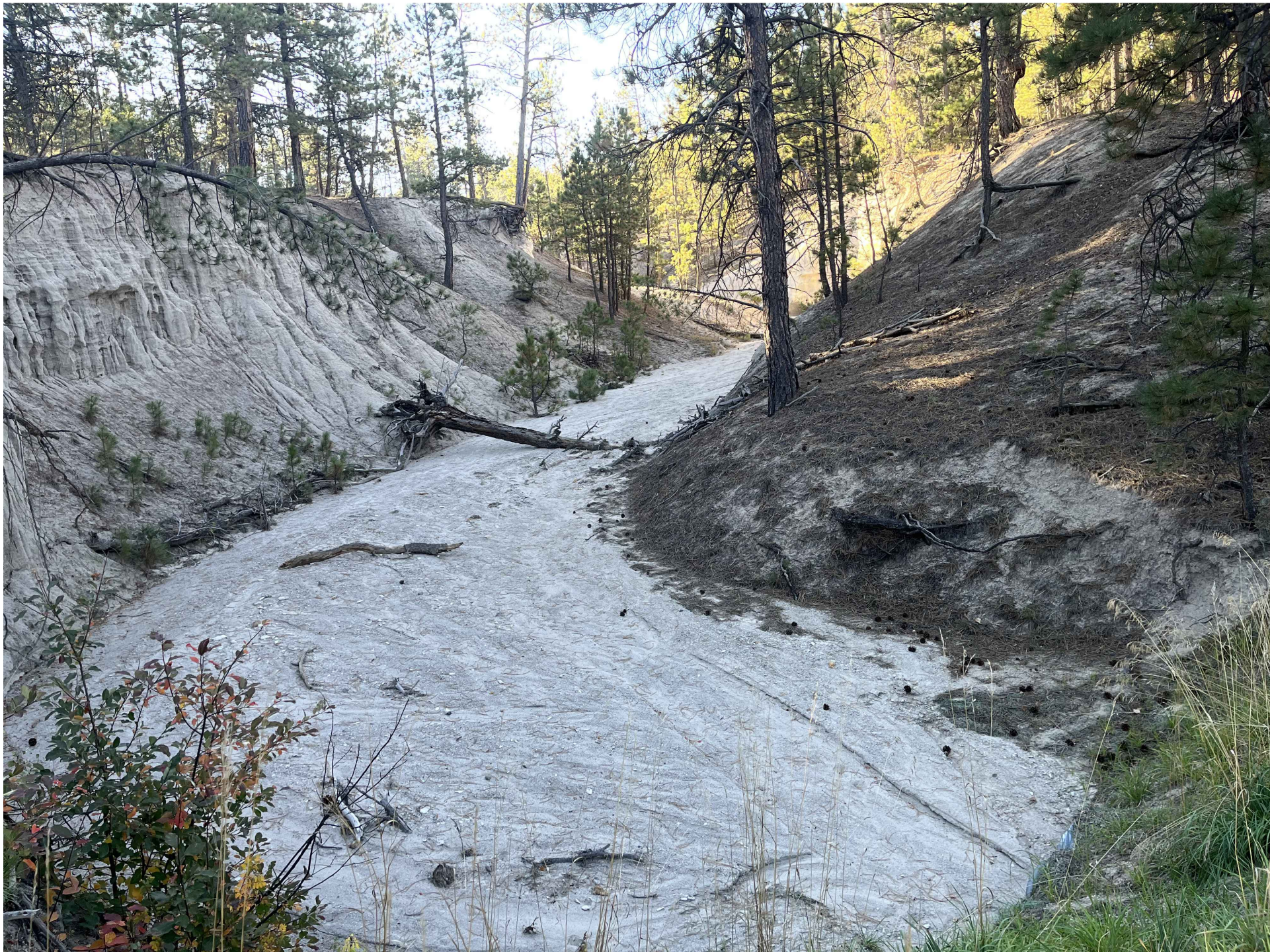
8. EXISTING TRIPLE 24' RCP CULVERT-UPSTREAM
