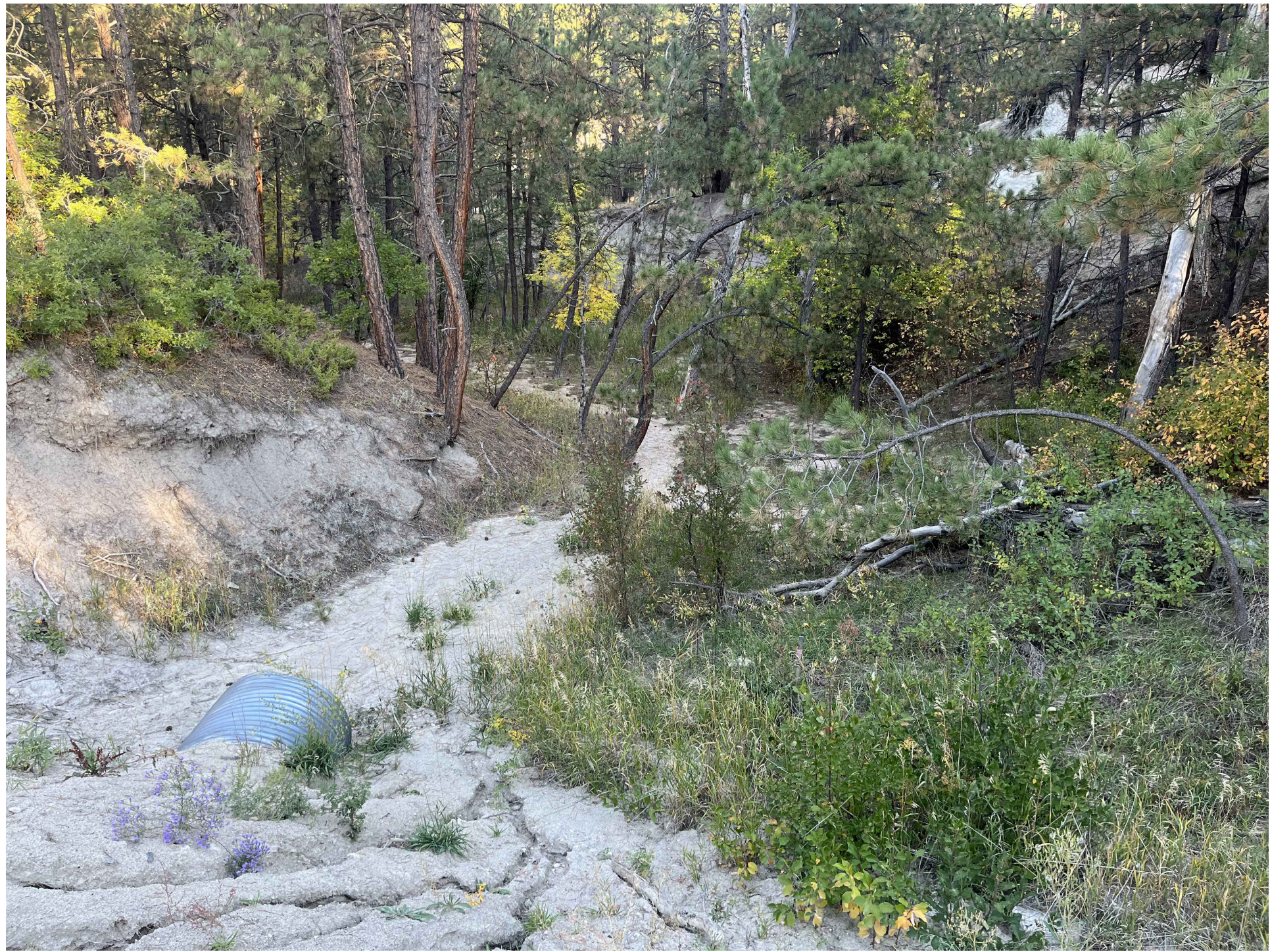
4. EXISTING 48" RCP CULVERT-DOWNSTREAM
