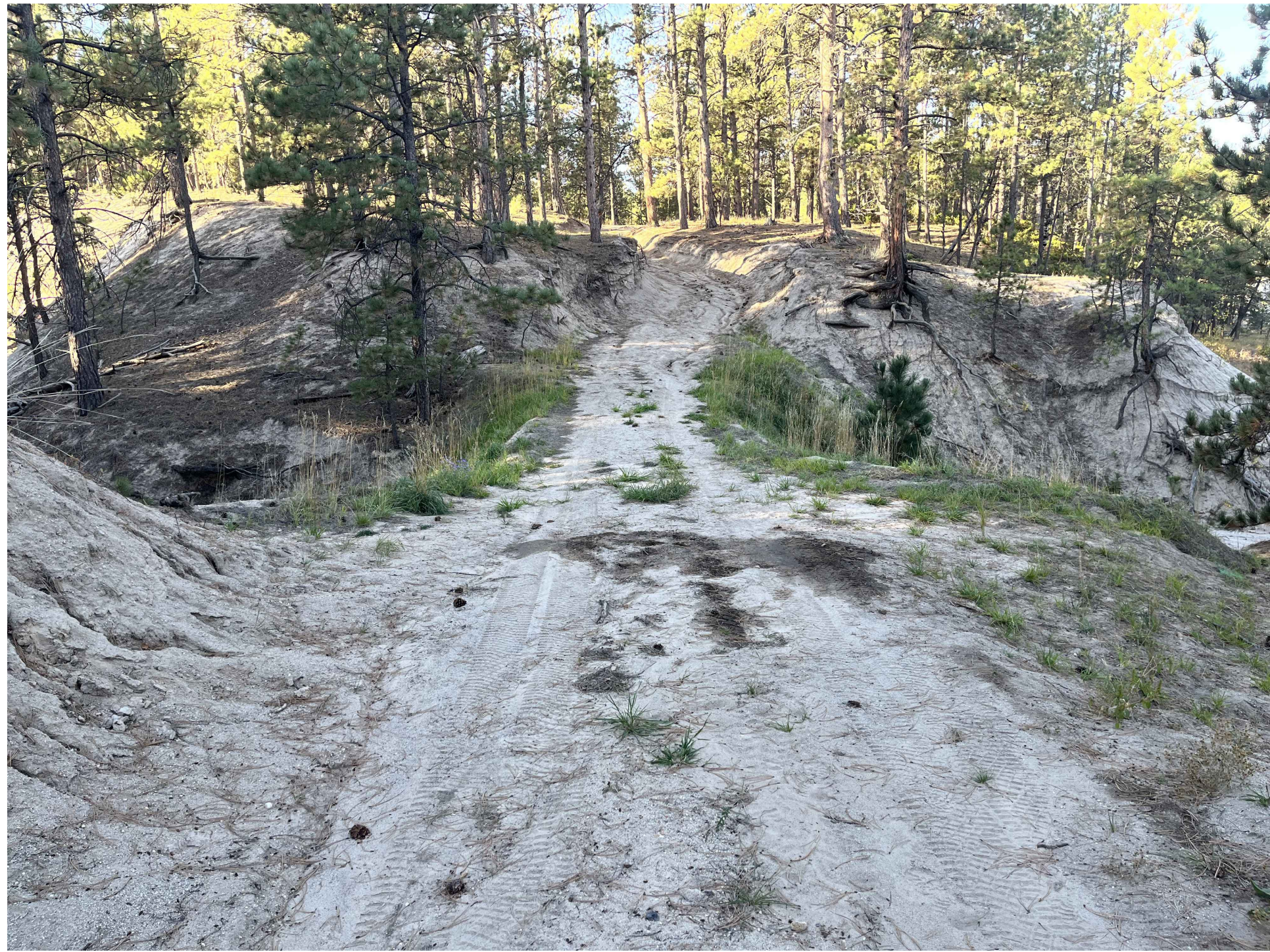
6. EXISTING TRIPLE 24" RCP CULVERT FROM ROAD
