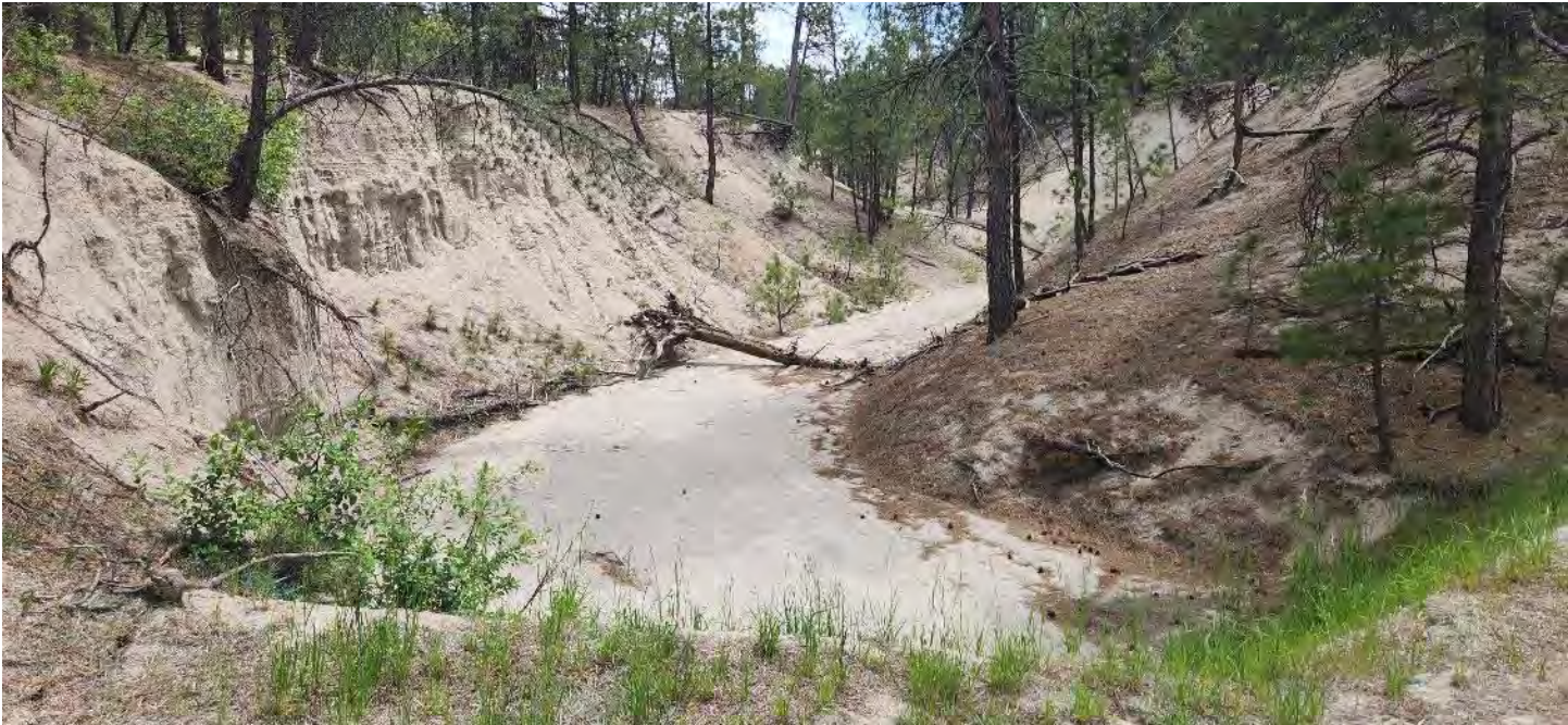
Photo Point 17 – View upstream of Drainage 3 from existing access road.
