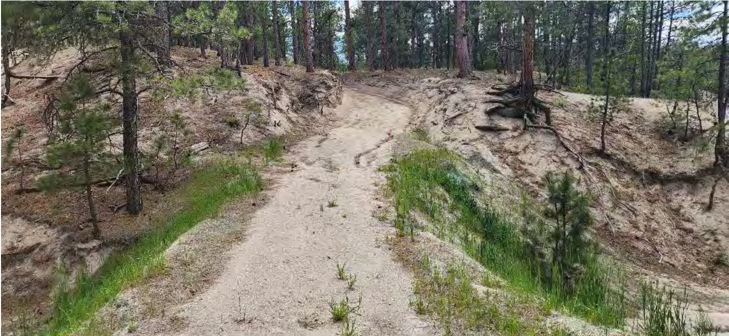
Photo Point 17 – View southwest (perpendicular to Drainage 3) of existing access road.
