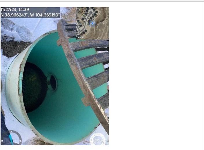
Photo 2: Missing restrictor plate on North and South Sand Filter Basins. Not installed as per Homestead 2 Sand Filter GEC Plans sheet 8 of 8.
