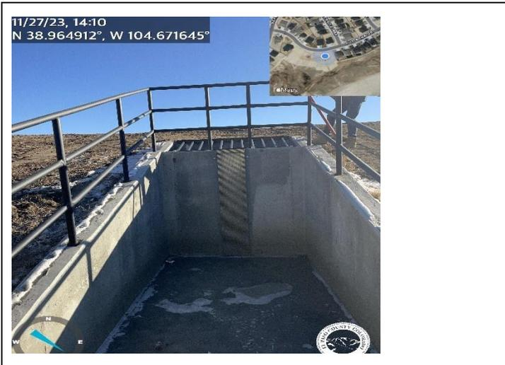
Photo 1: Well screen has been installed, but it is the wrong orientation. Note this is acceptable on the as-builts.
