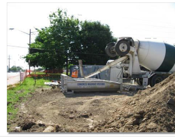
Photograph CWA-2. Prefabricated concrete washout. Photo courtesy of CDOT.
