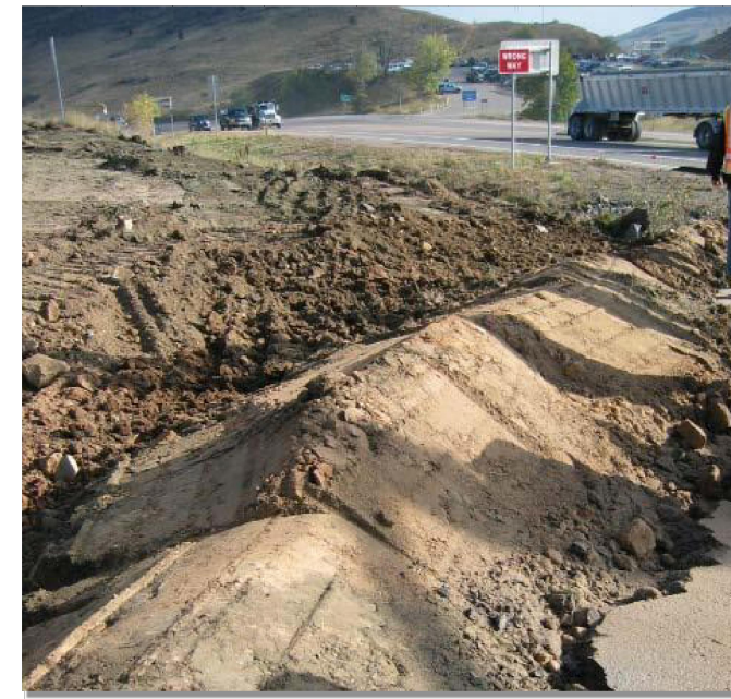
Photograph ED/DS-1. Example of an earth dike used to divert flows at a construction site. Photo courtesy of CDOT.
