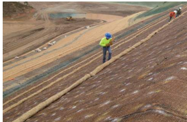
The RollMax TRMs are installed in a one-step operation directly over the prepared seedbed saving time and money and ensuring the highest level of erosion control and vegetation reinforcement.
