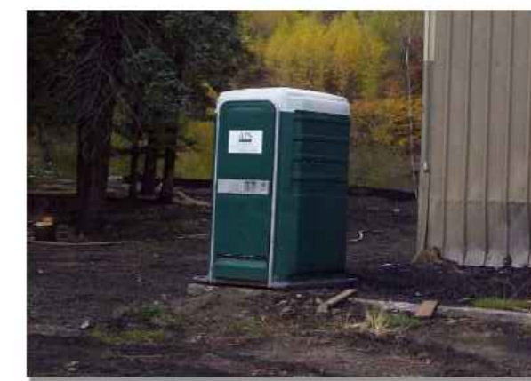
Photograph GH-3. Locate portable toilet facilities on level surfaces away from waterways and storm drains. Photo courtesy of WVE.
