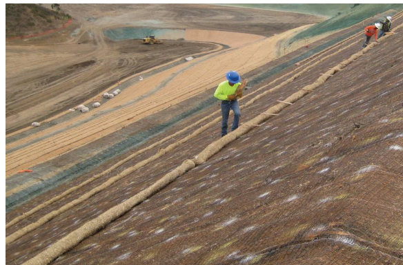
The RollMax TRMs are installed in a one-step operation directly over the prepared seedbed saving time and money and ensuring the highest level of erosion control and vegetation reinforcement.
