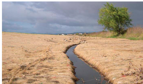
The EroNet temporary ECBs are designed to provide immediate erosion protection and vegetation establishment assistance, and then degrade after the vegetation is mature enough to permanently stabilize the underlying soil. Both short-term and extended-term ECBs are available.
