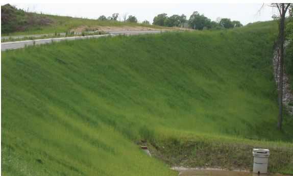
The EroNet temporary ECBs are designed to provide immediate erosion protection and vegetation establishment assistance, and then degrade after the vegetation is mature enough to permanently stabilize the underlying soil. Both short-term and extended-term ECBs are available.
