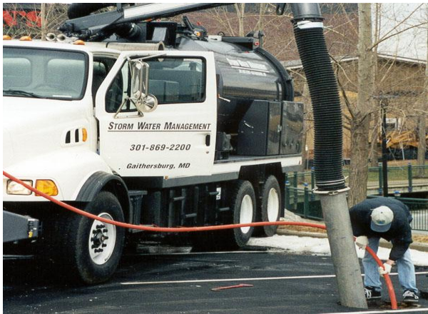
Figure 5: Vacuum truck and high pressure hose
