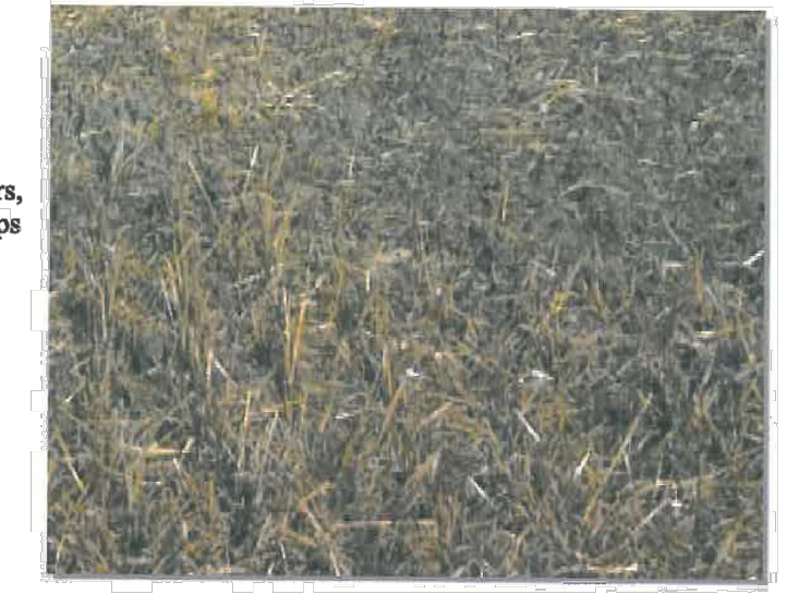
Photograph MU-1. An area that was recently seeded, mulched, and crimped.
