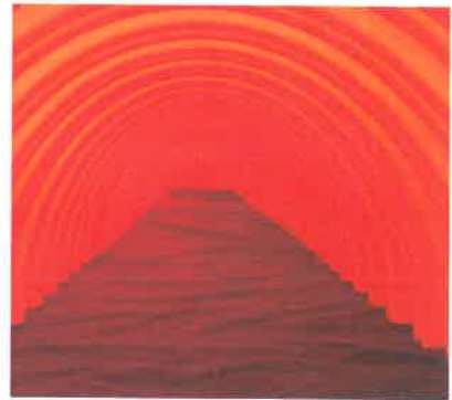
Looking down the Isolator Row from the manhole opening, woven geotextile fabric is shown between the chamber and stone base.
