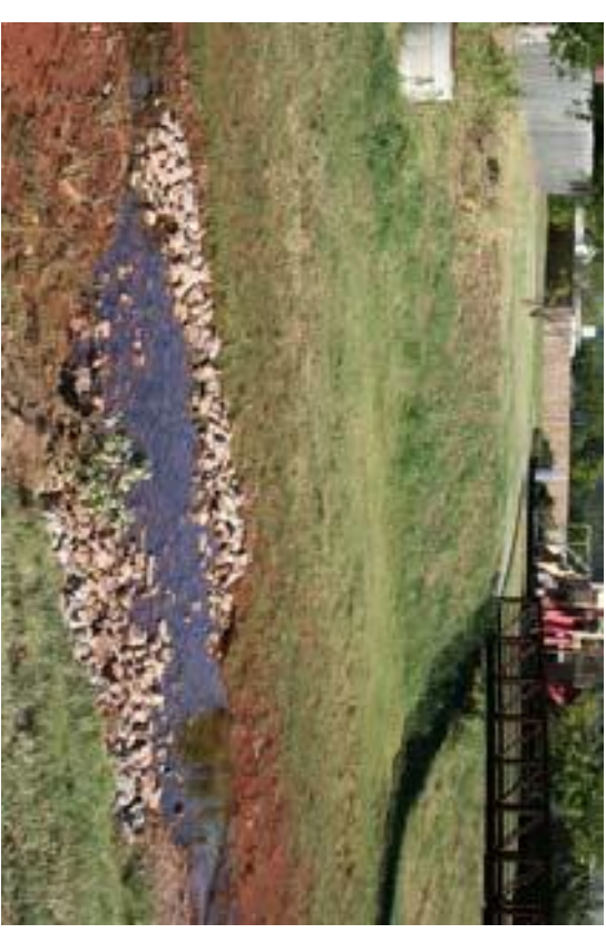
CONSTRUCTED RIFLE DROP STRUCTURE
