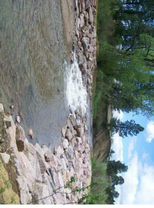
CONSTRUCTED GROUDED SLOPING BOULDER DROP STRUCTURE
