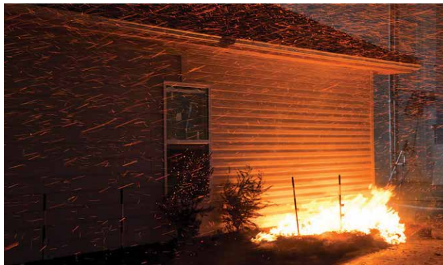
Flying embers are the most common source of home ignition during wildfires. Preparing homes for their impact is critical. Embers can ignite leaf litter in gutters and on roofs, as well as shrubs and mulch at the base of the house, as seen in this controlled ember shower experiment. Photo: Insurance Institute for Business & Home Safety
