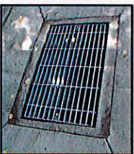
COOT Type C Grate (Close Mesh)
