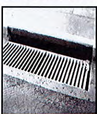
Directional 45-Degree Bar Grate
