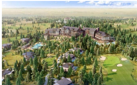
Figure 18-A luxury resort hotel is planned on FHN that will serve as a major tourism destination.
