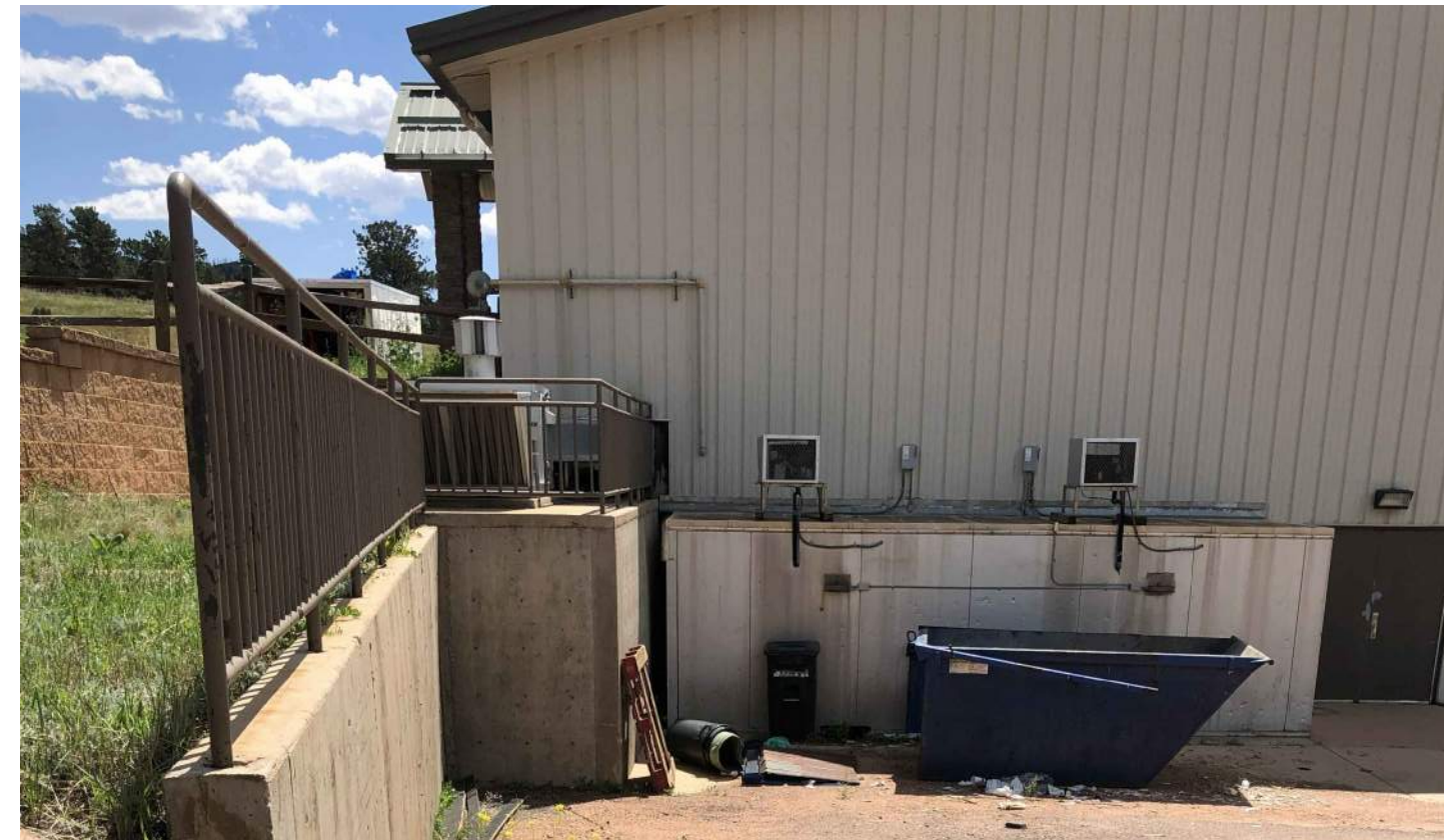
WEST ELEVATION (NO WORK BEING DONE)
