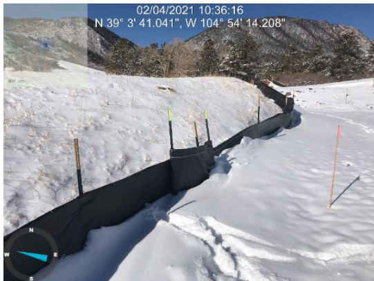
Wireback silt fence maintenance has occurred along end of F5.
