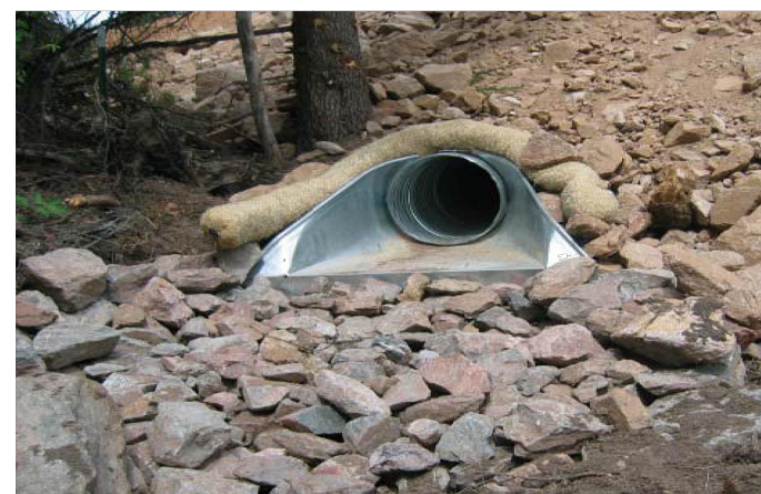
Photograph TOP-1. Riprap outlet protection.
