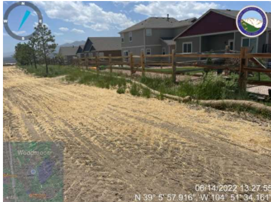
Disturbed areas have been temporarily stabilized and seeded.
