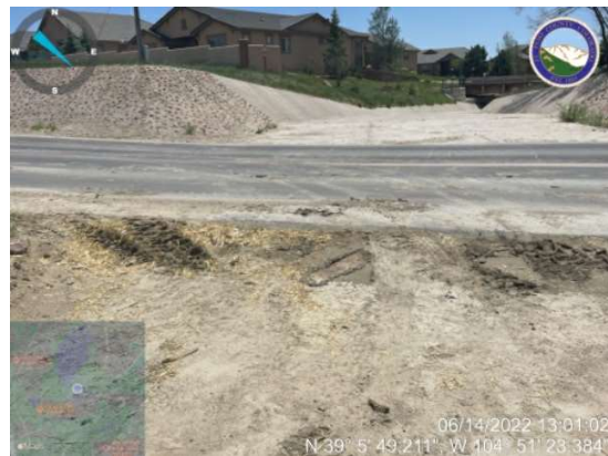
Sediment tracking near Lake Woodmoor dam occurring on Lake Woodmoor Drive. Increase street sweeping program.
