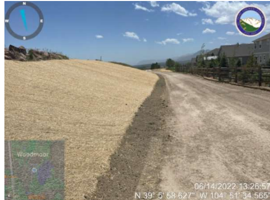
3:1 slopes that were disturbed have been matted with ECB.
