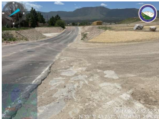
Sediment tracking near Lake Woodmoor dam occurring on Lake Woodmoor Drive. Increase street sweeping program.
