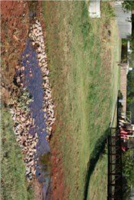
CONSTRUCTED RIFFLE DROP STRUCTURE
