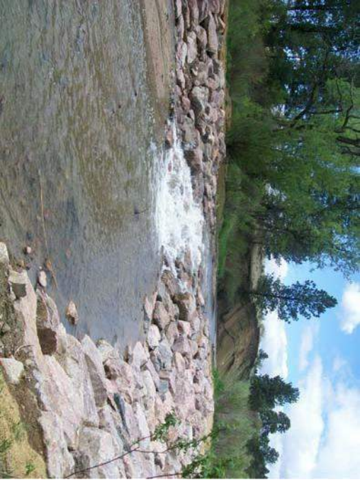
CONSTRUCTED GROUDED SLOPING BOULDER DROP STRUCTURE
