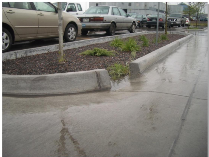
Photograph B-4. The curb cut shown allows flows to enter this rain garden while excess flows bypass the facility.
