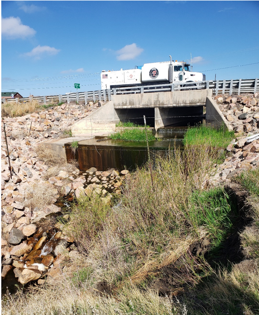
Existing 2-12'H x 4.83' W box culverts under Highway 24
