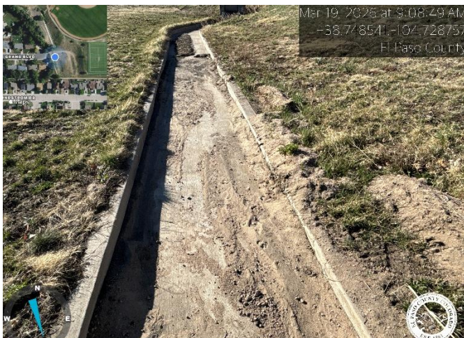
Photo 3: Remove sediment from Trickel Channel.
