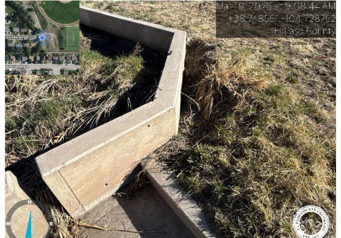
Photo 2: Repair Forebay erosion and repair erosion.
