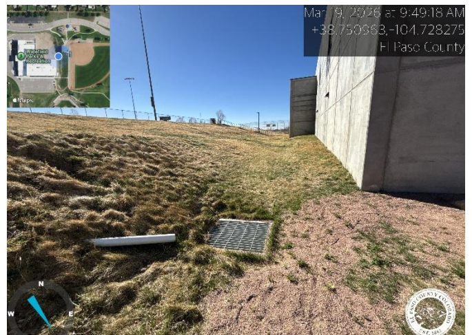
Photo 12: Inlet northeast area. No action needed.
