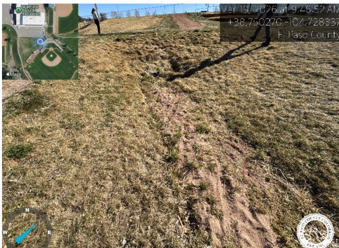
Photo 11: Southeast of parking area. Monitor erosion for future problems.
