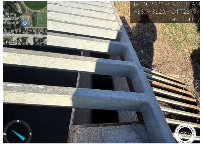
Photo 6: Add concrete crossmember to top of Outlet Structure.
