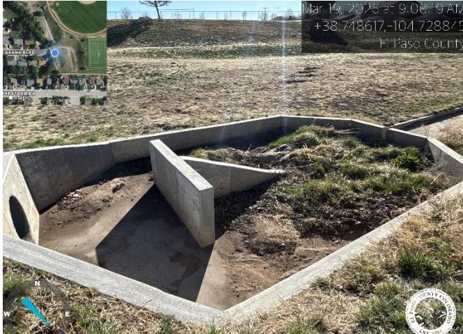
Photo 1: Remove sediment from Forebay.
