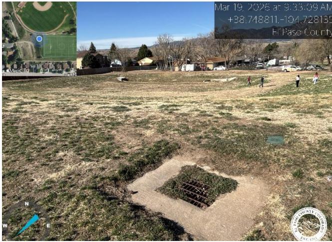
Photo 9: 2 Inlet drains. East side of pond, show on as-builts.
