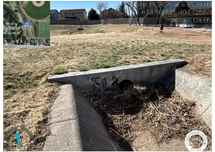
Photo 10: Clean out Drainage Ditch before pond.
