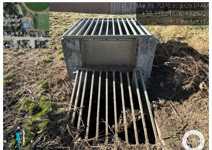
Photo 4: Clean Trash Rack and repair lock mechanism.
