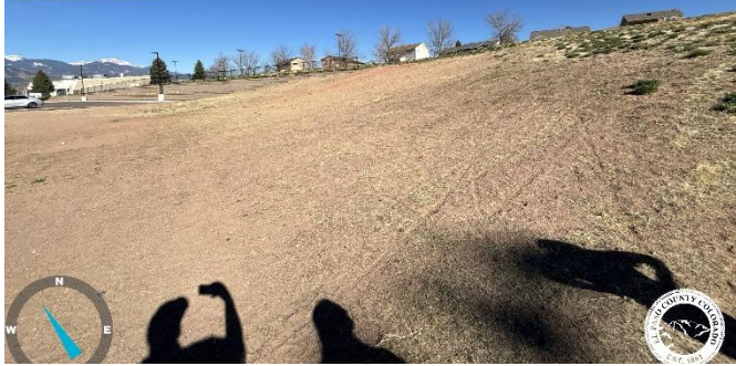
Photo 13: Northeast of building. Vegetation has not met requirements. Update Pond Calcs and As Builts to show this impervious area or stabilize.
